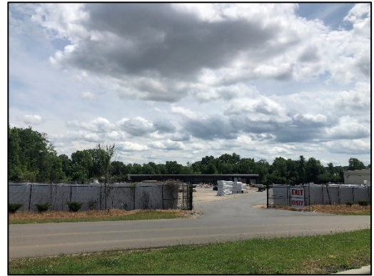
BMC Building Materials bordering the site to the west
